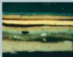
85. Paint sample from the exterior of one of the results of the partitions of the women's galleries, accompanying the stratigraphic study of fig. 80; [magnified 100x in incident polarized light]. The first grey finishing stages are identifiable at the bottom, followed by a greenish stage, a light blue stage (with every large grain of blue pigment), and three faux wood stages. The faux wood stage can be identified by the dark brown covering layers. The top layer is the present-day turquoise green finish.
